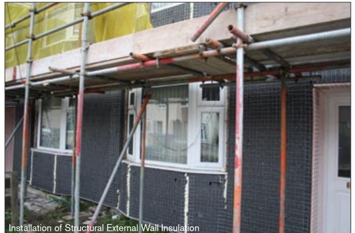
Installation of Structural External Wall Insulation
