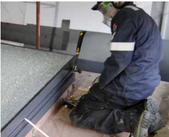
Part Q security testing process on Visionvent opening glass rooflight.
