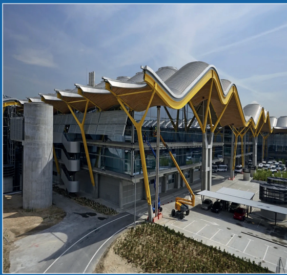
MADRID Barajas International Airport Source: Shutterstock
