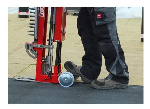
EJOT's ECOset HTK installation tool automates the fixing of the HTK 2G 50 tubewasher / fastener combination system. That means super-fast installation, better roof-top safety and greater all-round efficiency. EJOT is the first manufacturer to offer a battery powered installation tool, eliminating electric cables and tripping hazards. An additional cartridge holder is available, allowing up to 50 extra Dabo® fasteners to be housed.
