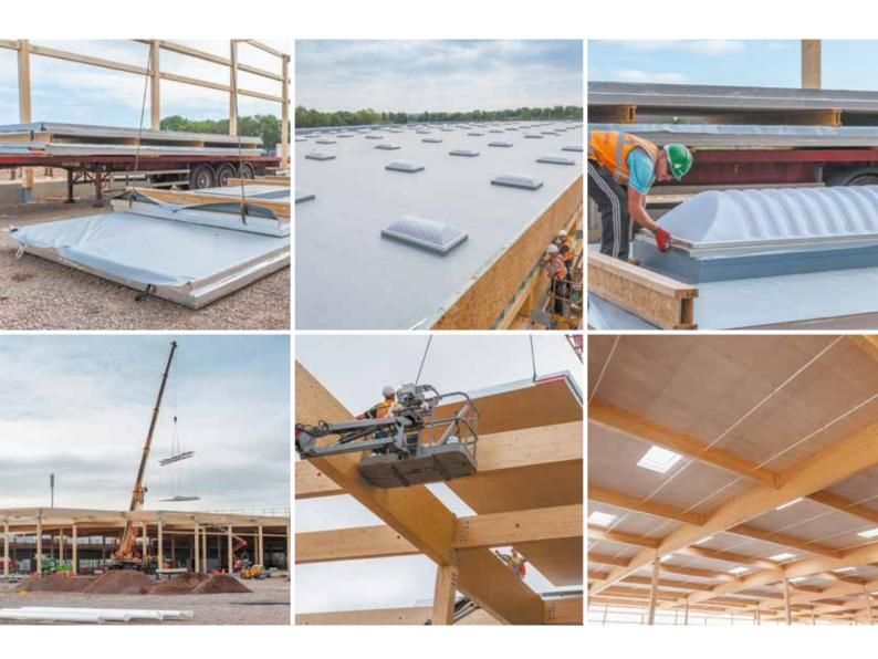
Pre-Fabricated, Long Spanning Roof Elements for Fast Track Construction
