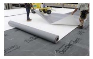
Independent ASTM D5635 puncture tests' indicated that thermoplastic membranes do not puncture as easily when 6.4 mm (1/4 inch) DensDeck® Prime Roof Boards are used as a cover board, as compared to no cover board or HD ISO cover boards.
