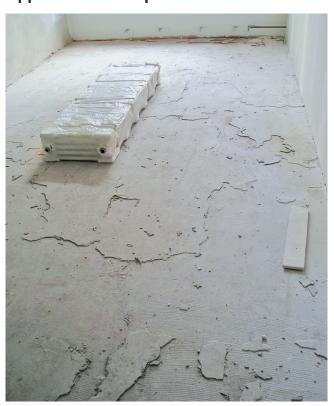
Old screeds with unstable adhesive and poorly adhering levelling compound layers can be renovated with UZIN NC 110 low-stress levelling compound.
