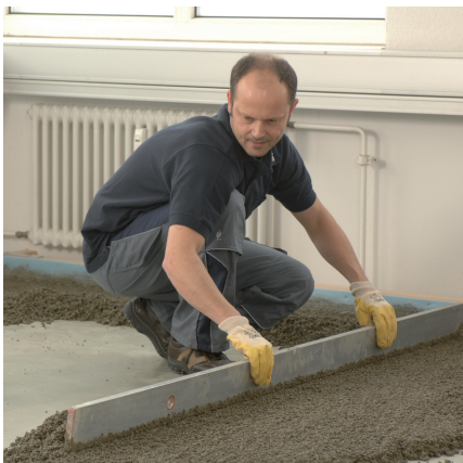
Application of the light smoothing mortar UZIN SC 914 Turbo
