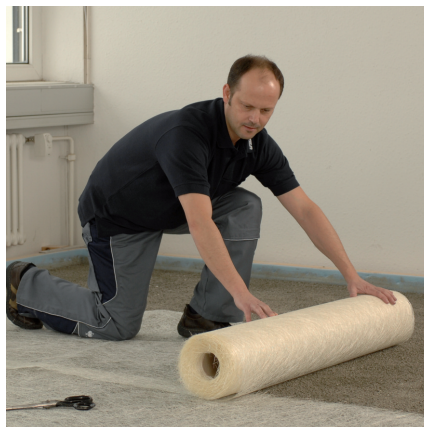
Installation of the renovation fleece UZIN RR 201
