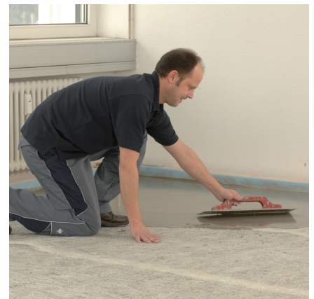
Application of the thin screed UZIN NC 195
