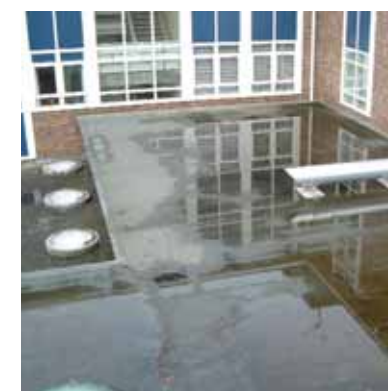
Ponding caused by poor design and maintenance
