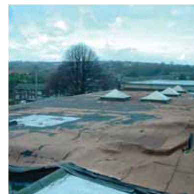
Wind damage resulting from poor design
